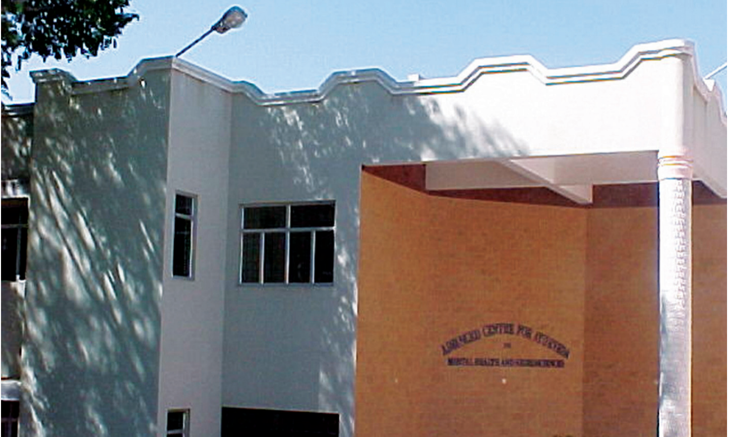
View of ACAMH & NS premises, Bangalore
